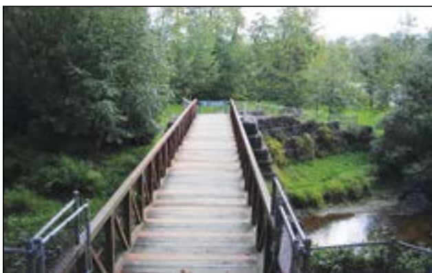
Al Borlin Park park is accessible by this footbridge from Lewis Street Park or by vehicle via Simons Road.
